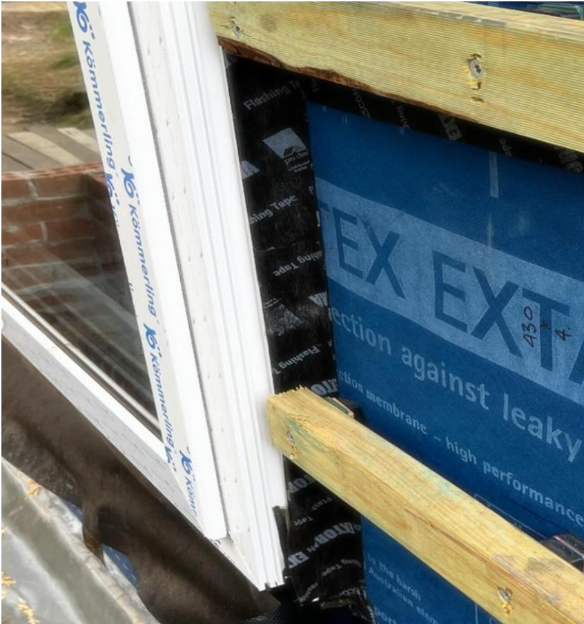
A window installed in the ventilation cavity
